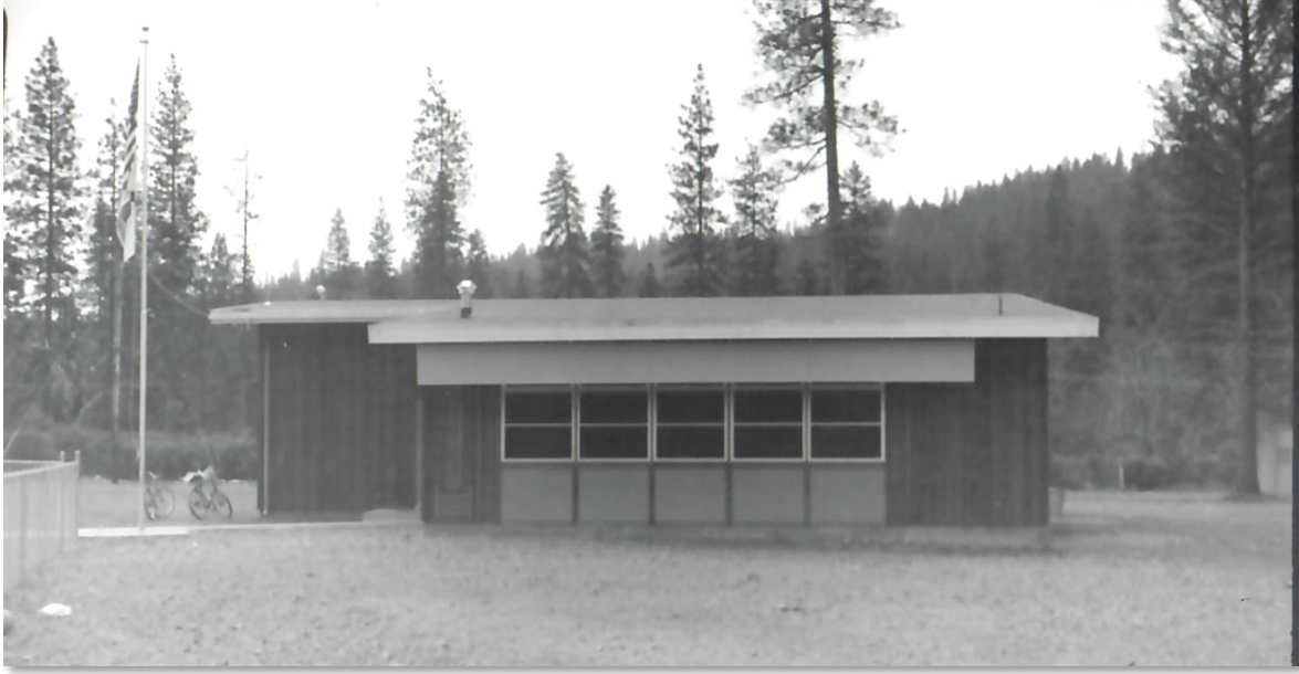
Ruth School Constructed in 1964, closed in 1969, and now the Ruth Community Church.
